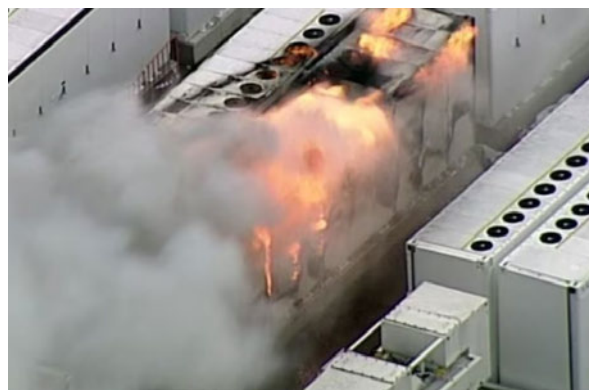
Figure 7: The starting fire plume at the Geelong BESS module (taken from web source: https://www.abc.net.au/news/2021-09-28/fire-at-tesla-giant-battery-project-near-geelong-investigation/100496688 , accessed June 2024).
